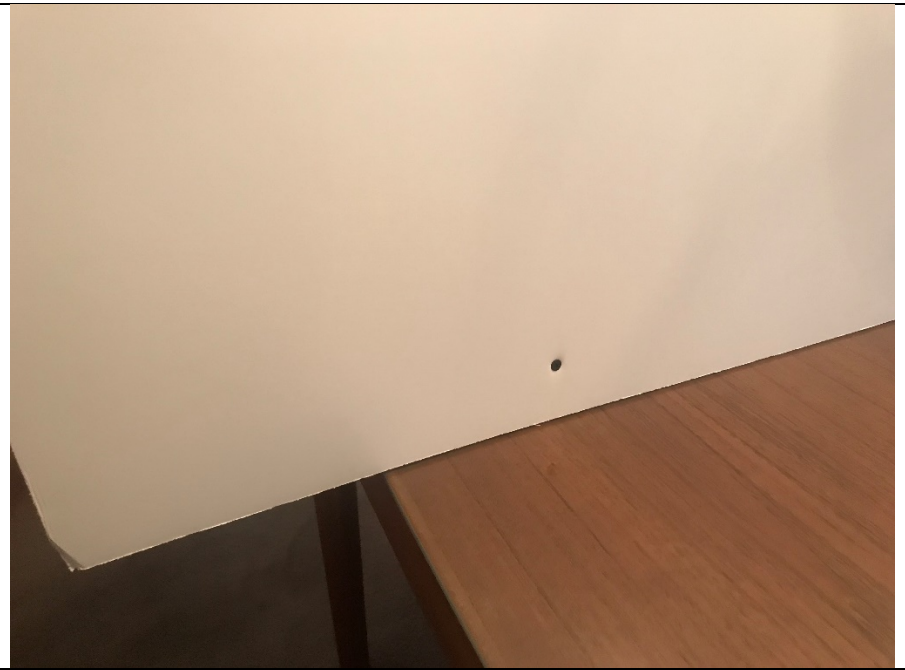
Single points from foam core board to wooden support behind (2 screws)
